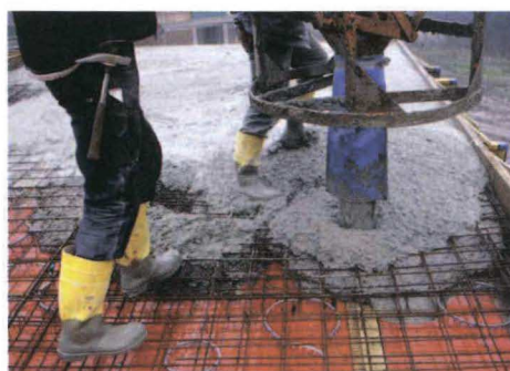
In-situ reinforced concrete being poured
