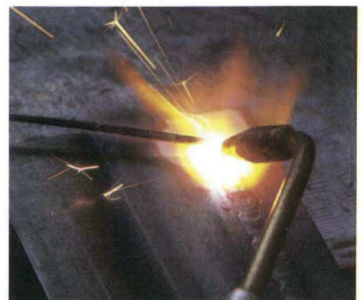
Gas welding using oxyacetylene
