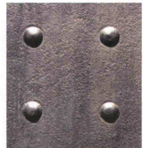
Solid rivets after installation
