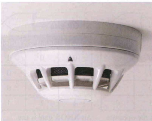
A smoke detector
